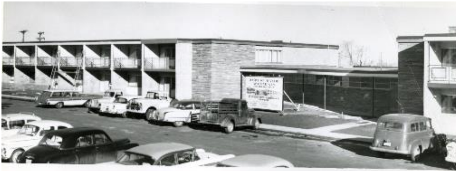
The finished Murchison apartments at the hotel complex. Carnegie Library for Local History/Boulder Daily Camera Collection.
