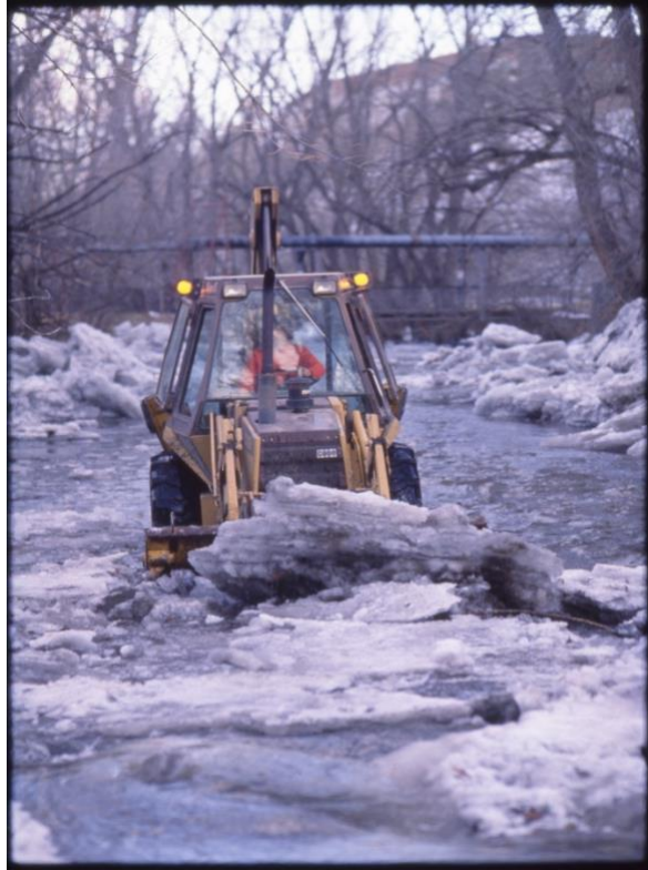
In January of 1991, Boulder Creek overflowed its banks spilling water onto the hotel's tennis courts and threatening nearby buildings including the tennis pro shop. Here, ice is removed from the creek. Carnegie Library for Local History/Boulder Daily Camera Collection.
